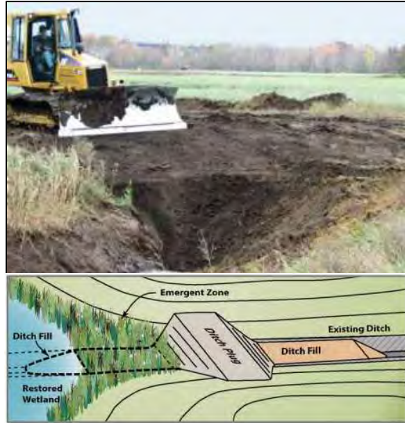
Figure 35 - Earthen lateral ditch plug concept and installation. Source: MN Wetland Restoration Guide, BWSR.
