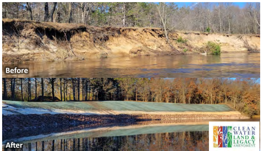
Photo: Downstream half of the project post-construction.
