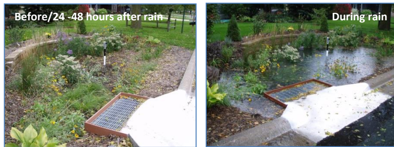
Figure 3: Rain garden before and during a rainfall event
