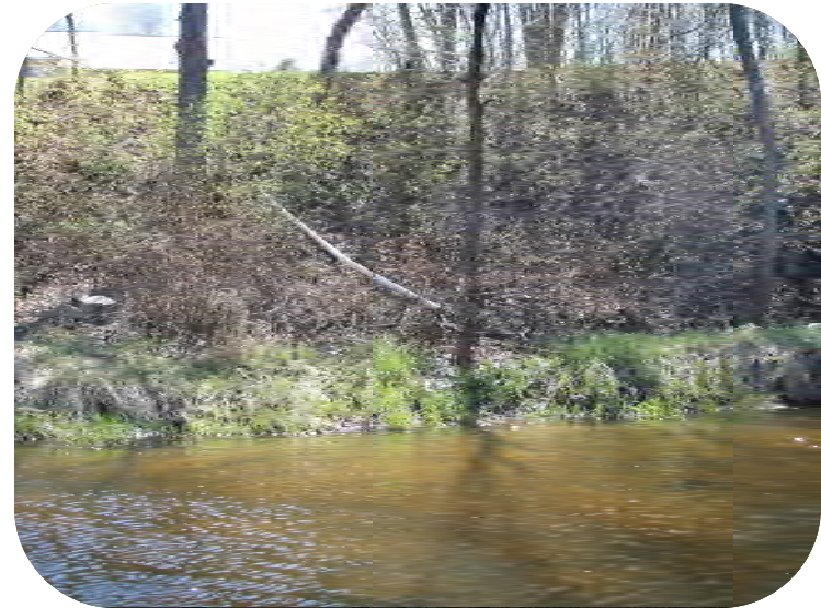
Photo 76 – Approx. 3 in. diam. PVC outlet near toe of slope with high flow and erosion.
