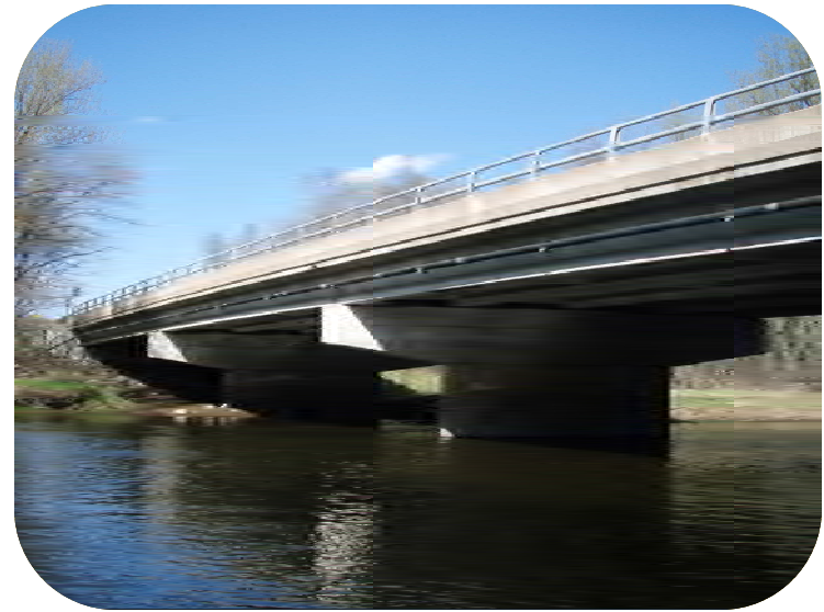
Photo 118 – County Road 7 bridge.
