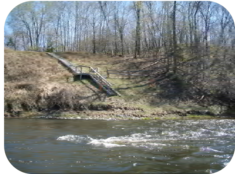
Photo 84 – Gas pipeline crossing. Also see Photo 85.
