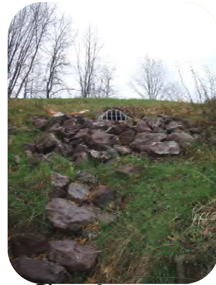
Photo 6 – Stormwater outfall. 20" dia FES
