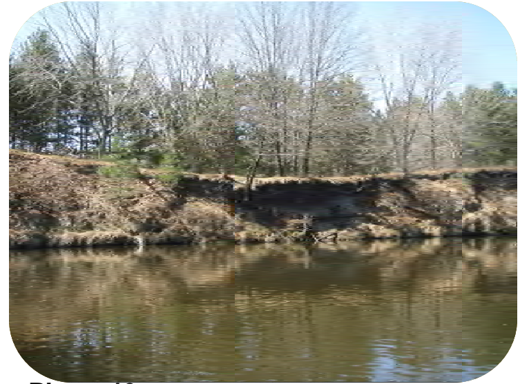
Photo 46 – Severe erosion. Also see Photos 47, 48, 49, 50, 51, 52, and 53.
