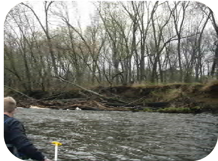
Photo 28 – Moderate erosion severity, approx. 50 ft. long. Low priority.
