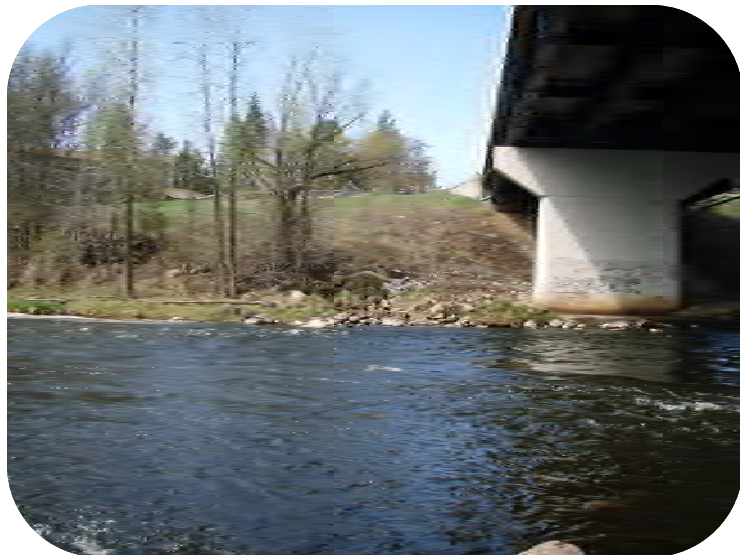
Photo 31 – Outfall with concrete water break and rock apron. Also see Photo 32.
