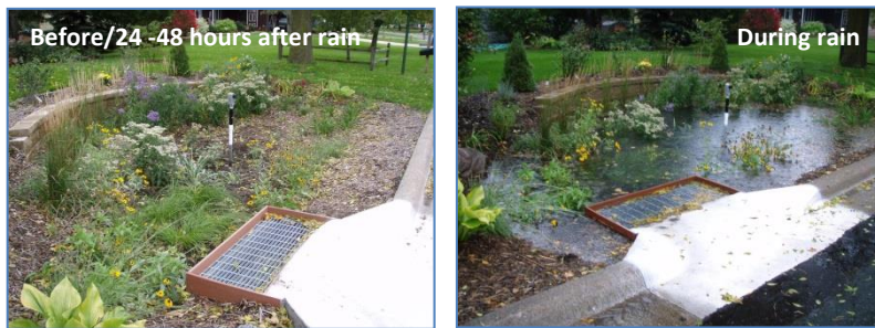
Figure 4: Rain garden before and during a rainfall event
