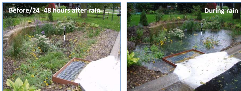
Figure 5: Rain garden before/after and during a rainfall event
