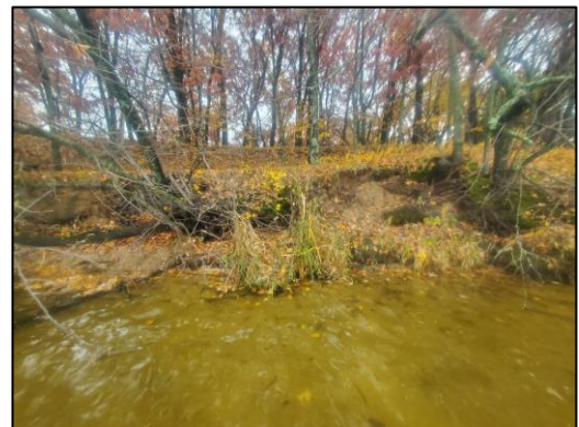
One of the 2024 lakeshore stabilization sites.
