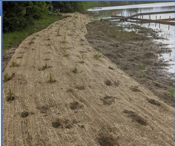
Project area. Installed July 2022.
