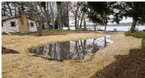
Stormwater pond rehabilitation—Martin Lake
