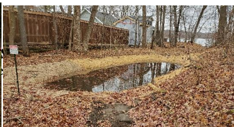
Stormwater pond rehabilitation—Martin Lake
