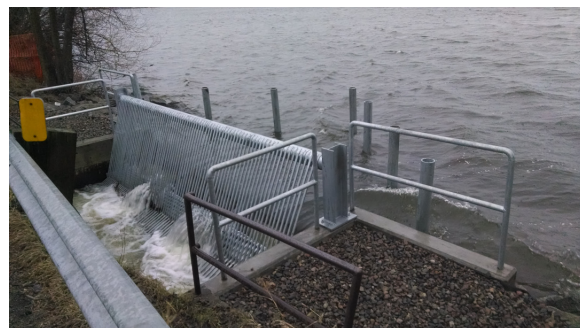
Martin Lake outlet (completed early 2016)
