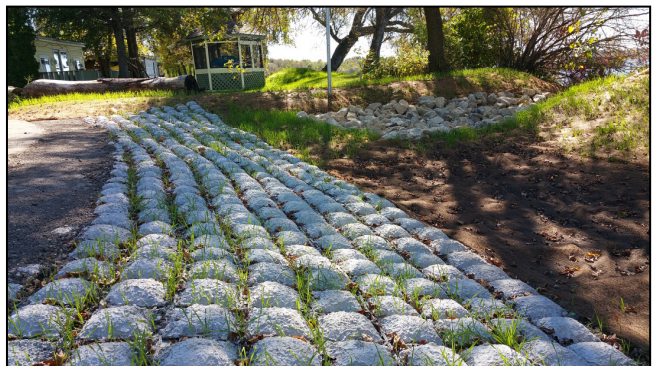
Lincoln Avenue stormwater stabilization.
